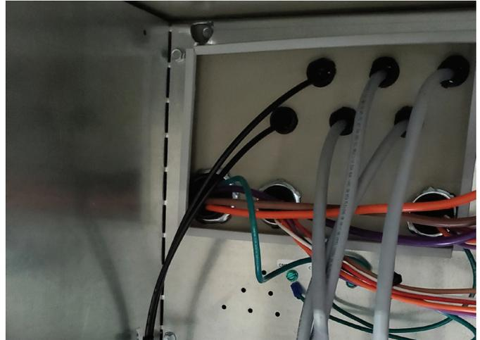
**Figure 54: Patch Plate with One Grommet Removed**
