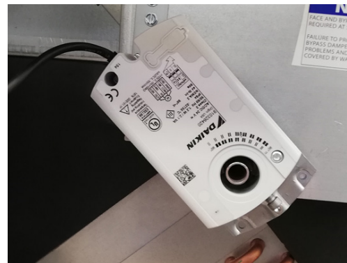
Figure 110: Face & Bypass Actuator
