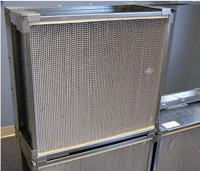
Figure 48: Properly Installed Filter Inside of the Frame
