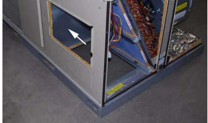
Figure 2. Non-Turbulent Airflow Area for Mounting
