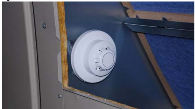
Figure 4. Junction Box and Smoke Detector Installed
