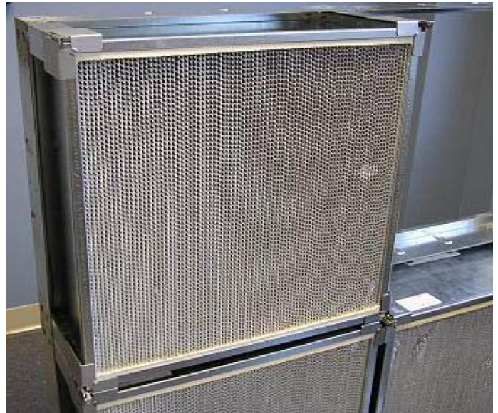
Figure 29: Properly Installed Filter Inside of the Frame
