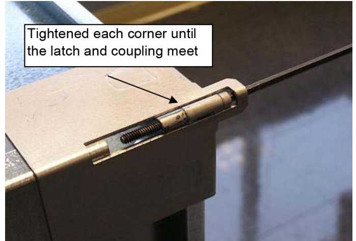
Figure 29: Properly Installed Filter Inside of the Frame
