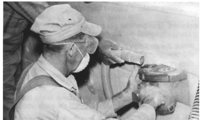
Figure 12: The interior wall opening is cut
