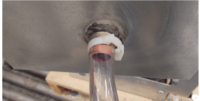
Figure 3: Connect PVC drain hose and clamp
