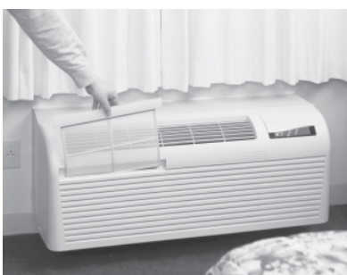
Figure 19. Room Air Filters
