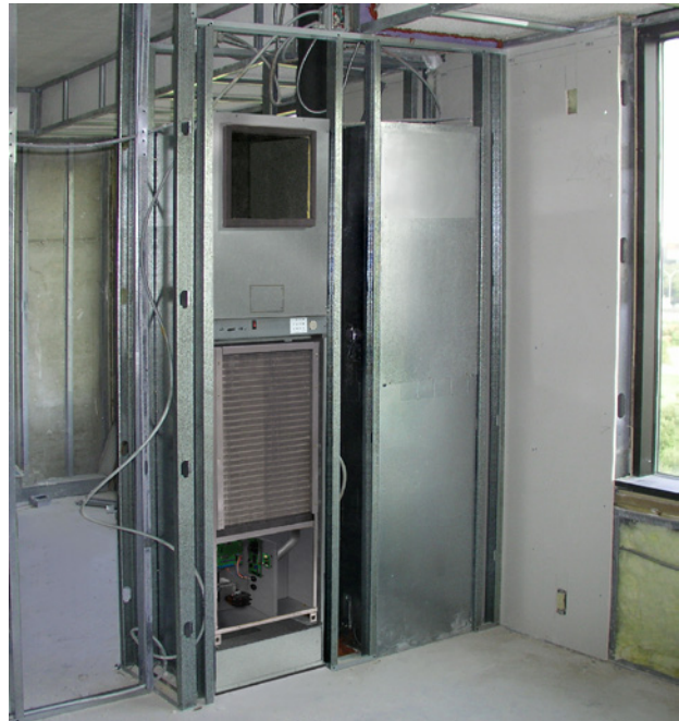
Figure 7: Typical side by side unit installation
