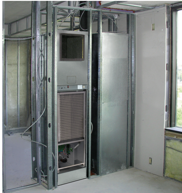
Figure 7: Typical side by side unit installation
