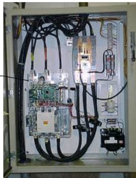
Wiring Connection on Starter for Optional Display
