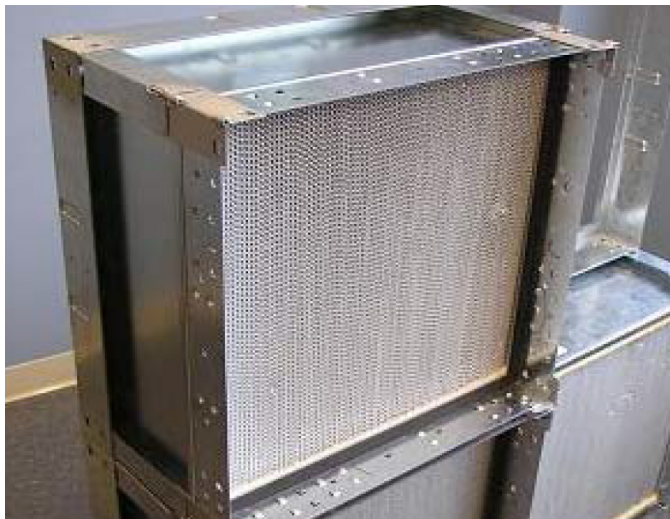
Figure 95: Properly Installed HEPA Filter
