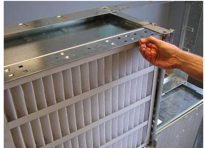
Figure 96: Installation of Prefilter Into Frame
