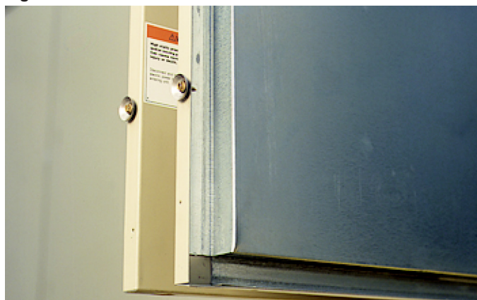
Figure 1: Full Double-Wall Construction
