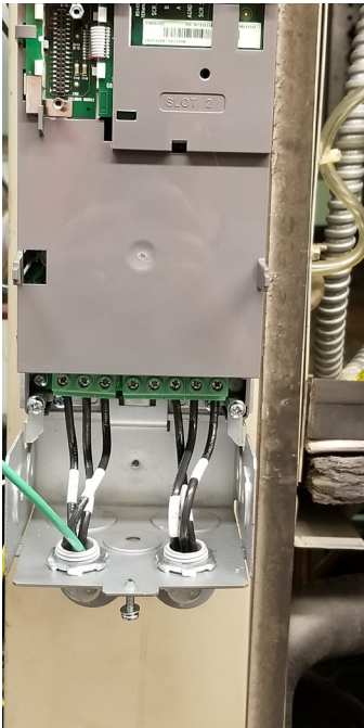
Figure 13: Actuators for Waterside Economizer
