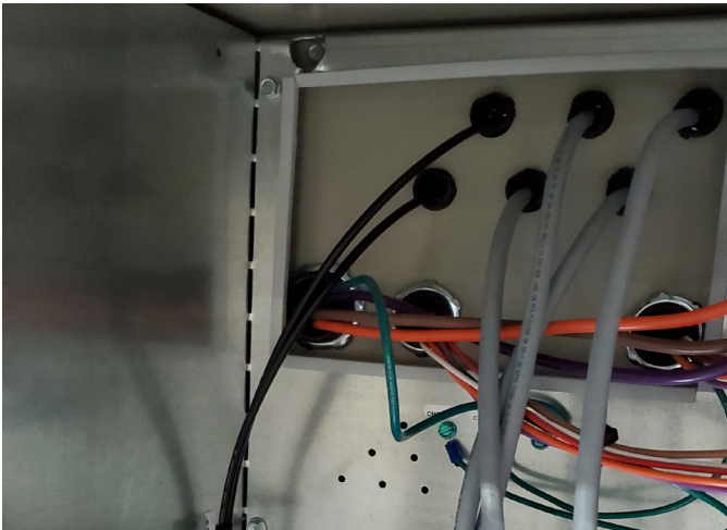
Figure 74: Rebel Applied Cabinet Knockouts
