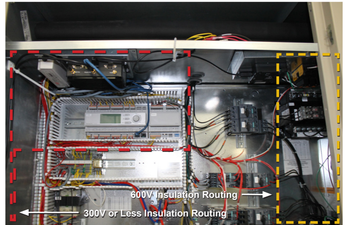
Figure 69: Typical Rebel Wire Routing
