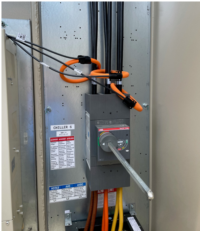
Figure 42: Installed Rogowski Coils
