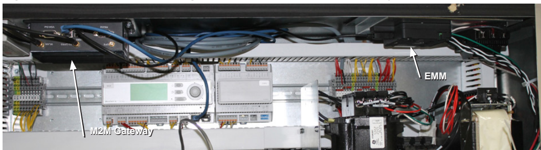
Figure 61: M2M Bracket Mounting Location – RoofPak (Generation 1 Gateway shown)
