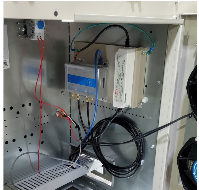
Figure 66: DPSA (Rebel Applied) Gateway Bracket Mounting Location
