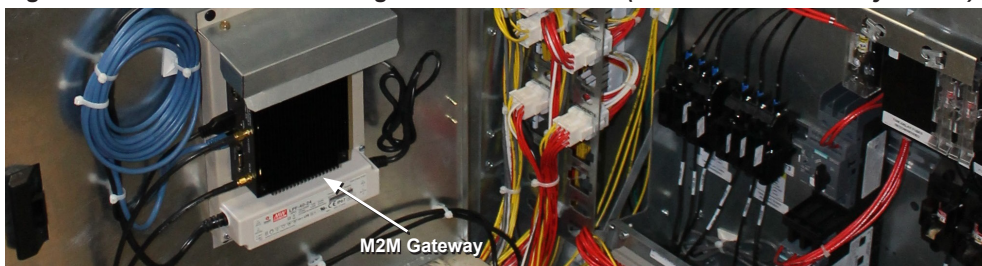
Figure 61: M2M Bracket Mounting Location – RoofPak (Generation 1 Gateway shown)
