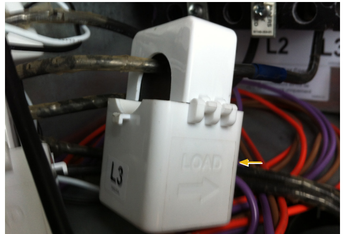
Figure 91: CT Installation
