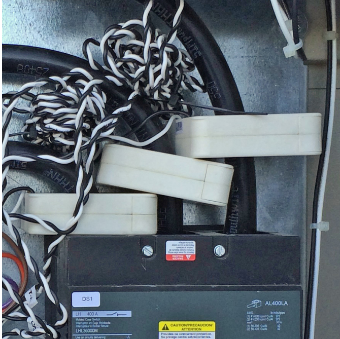
Figure 49: CT Installation
