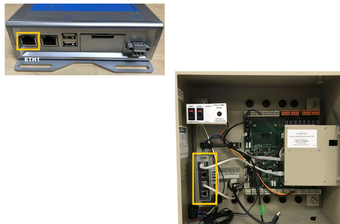
Figure 28: M2M Gateway Connection to WME Gen 1 Chiller (Generation 2 Gateway)
