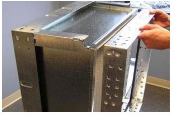
**STEP 6:** Place a latch so that the 2 tabs of the latch overlap the prefilter frame on each side of the corner. Slide the latch inside of the leg extension and align the latches' cap screw with the threaded coupling on the end of the leg extension and tighten using the hexkey. See Figure 28.
