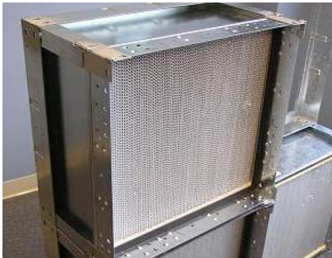
Figure 30: Properly Installed HEPA Filter
