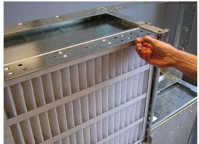
Figure 31: Installation of Prefilter into Frame
