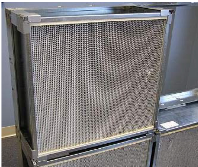
Figure 25: Properly Installed Filter Inside of the Frame
