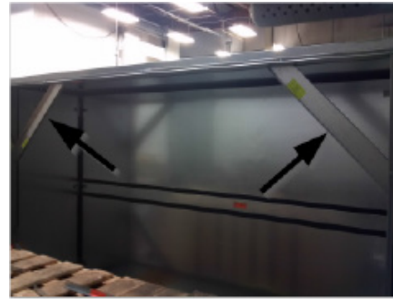
Figure 5: Shipping Braces
