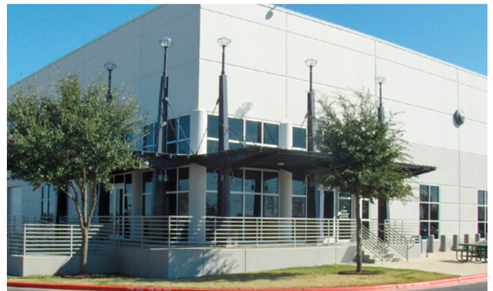
Waste Management data center facility, Austin, Texas
