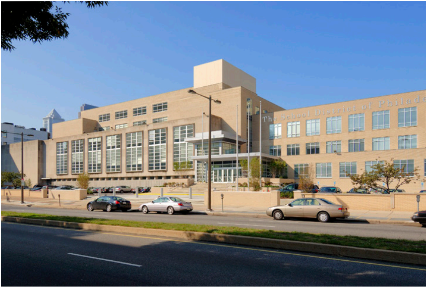
Self-contained air-conditioning systems at the School District of Philadelphia Education Center meet project requirements of low installed and operating costs and low maintenance.
