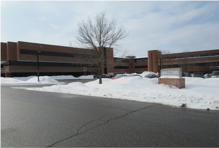
Vermont Information Processing's three-story building contains office space as well as a data center located on the third-floor.
