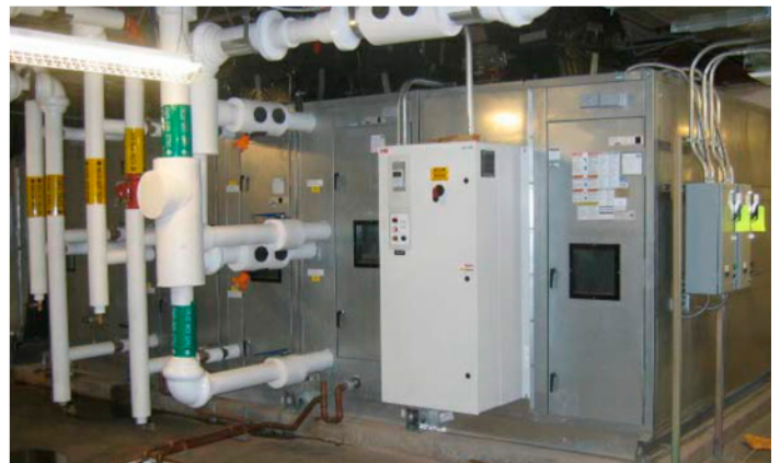
Four Daikin Vision indoor air handlers with energy recovery coils recover energy from the exhaust air stream and use it to pre-treat the supply air stream, helping to save on ventilation and energy costs.
