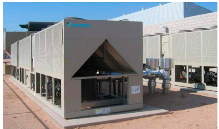
Daikin air-cooled screw compressor chillers deliver up to 14 EER at part load and use HFC-134a refrigerant with no ozone depletion or phase-out date.
